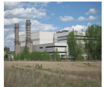
Xcel Energy’s High Bridge Plant Located in St. Paul, MN
