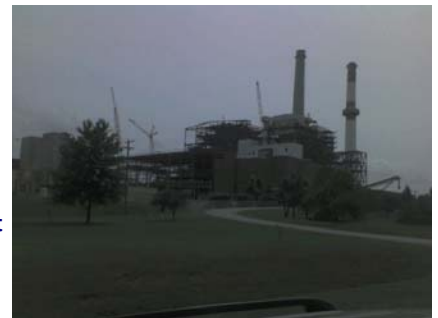
Southwest Power Station Owned and Operated by the City Utilities.
